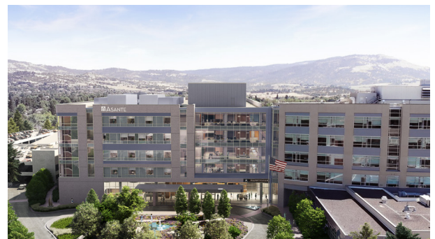
The new critical care beds will be housed on the third and fourth floors of the patient pavilion.
