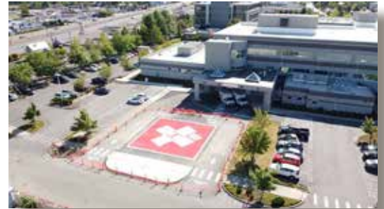
The new helipad, behind the ED.
